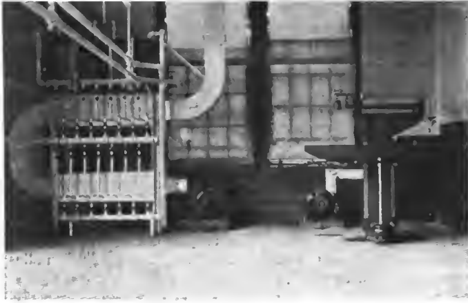
VIEW OF THE SECTIONAL RADIATOR AND BLOWER.
